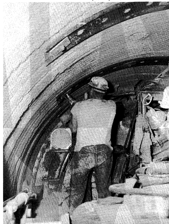
Figure 48: Workman tightening the nut on a rock bolt that holds a steel strap inside a mole-excavated tunnel. Laser beam target at left is used to guide steering of mole.
