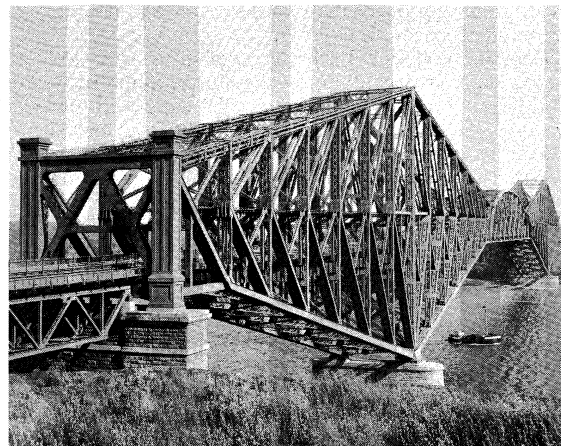
Figure 15: Quebec Bridge across the St. Lawrence River. The steel cantilever railroad bridge, spanning 1,800 feet, was completed in 1918.
