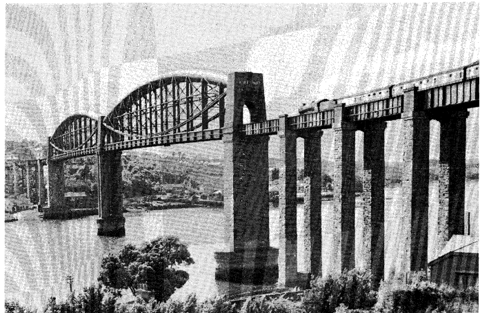
Figure 11: Royal Albert Bridge over the Tamar at Saltash, Cornwall. The designer, Isambard Brunel, employed a wrought iron cylinder 35 feet in diameter for the central pier in this innovative design of 1855–59.
