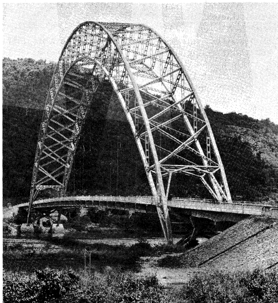
Figure 21: Adomi (formerly Volta) Bridge in Ghana, completed in 1956. This steel arch bridge utilizes high-strength friction-grip bolts at the connections between the chord members.
